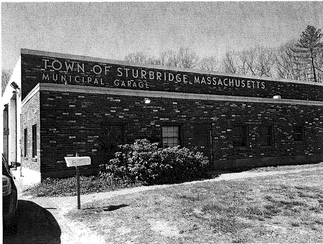
Figure 2: The main building on the site houses DPW administration, maintenance and storage bays. The public entrance is in the center of the photograph.
