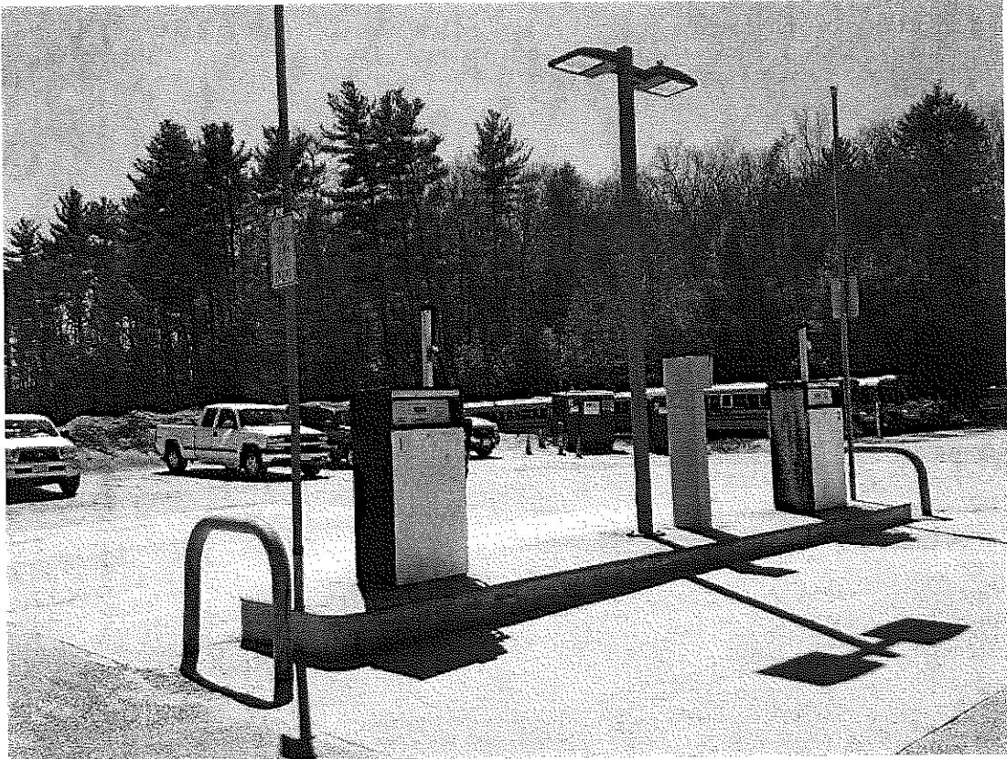
Figure 7: The existing fueling island is in good repair although dispensers will need to be replaced.
