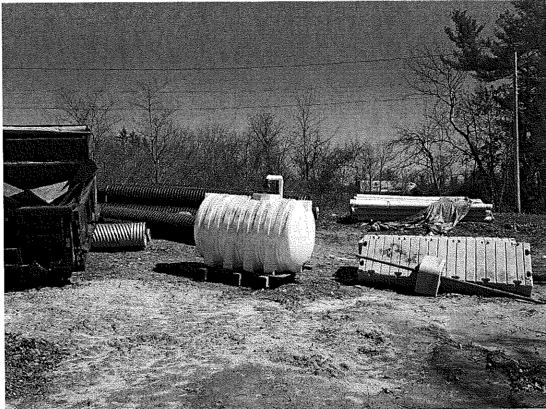
Figure 9: The area south of the Salt Shed is used for storage of drainage structures and conduit.
