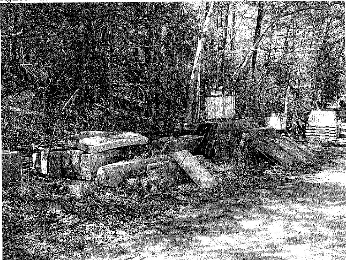
Figure 10: Areas for stockpiling of various roadway materials line the interior access roads.
