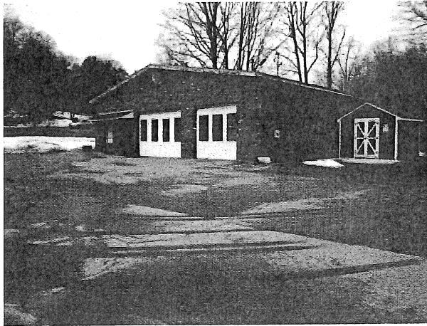
Photo No. 1. Front of building, facing northwest
