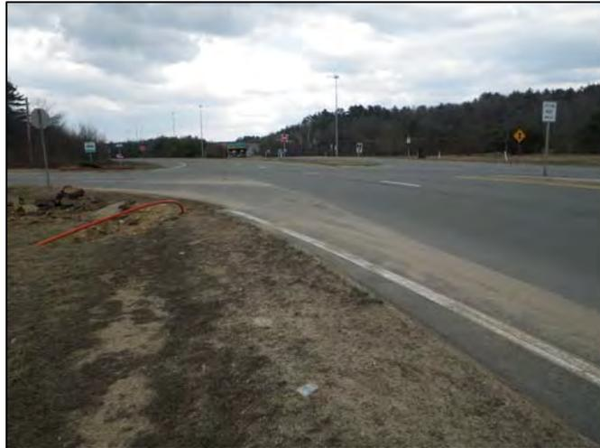
*Route 20 & New Boston Road: Drivers have difficulty entering Route 20 safely from New Boston Road due to the long crossing width and vehicle speeds on Route 20.*
