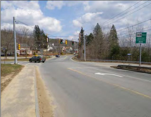
Sidewalks are located on the northeast and northwest corners of the intersection. No sidewalks are located on the southeastern or southwestern portions of the intersection as guardrail protects the Main Street (Route 20) from the steep embankment to the south. A marked crosswalk is located across the north leg of the intersection but is not accompanied by pushbuttons or pedestrian signals.
